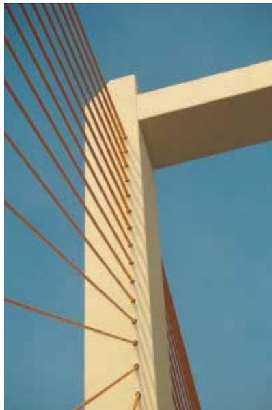
**The John James Audubon Bridge deck is supported by 136 parallel-strand stay cables arranged in a traditional semiharp pattern.**
