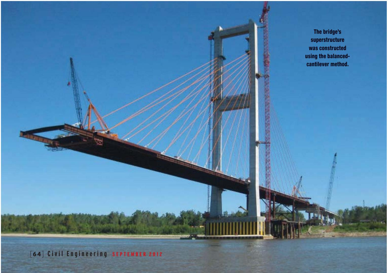
**The bridge's superstructure was constructed using the balanced-cantilever method.**
